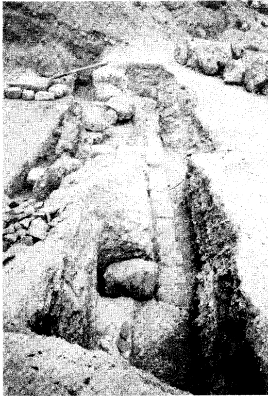
Foundations of the pylons in TT148
